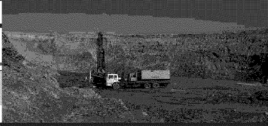
Drilling at Beta's expansive pit floor in preparation for mining
