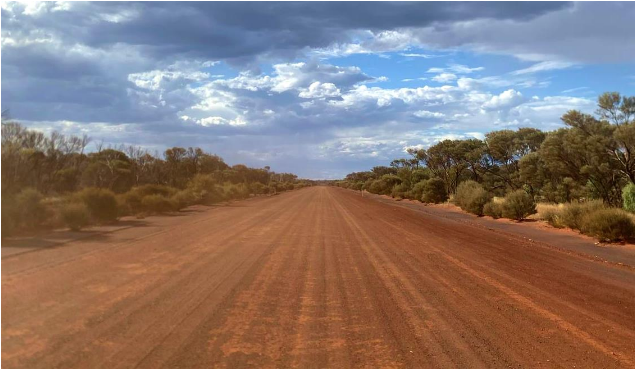
Figure 4: Jasper Hills private haul road – remedial works near completion
