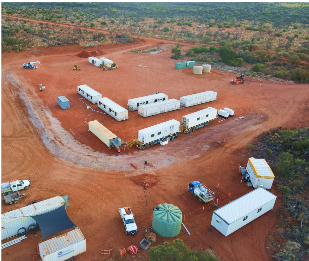
Figure 3: Site establishment underway
