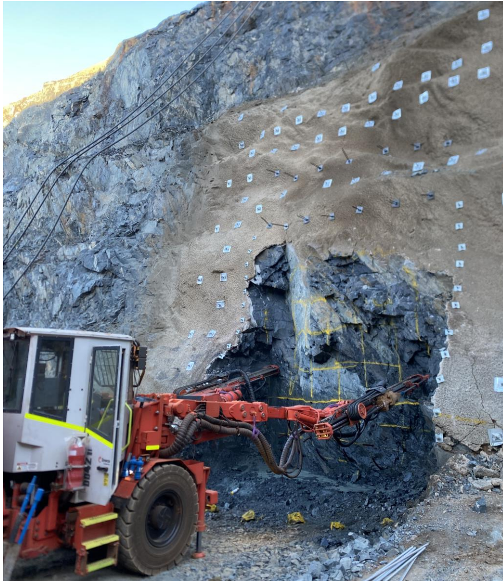
Figure 3 - Twin boom jumbo boring ahead of firing the next development cut
