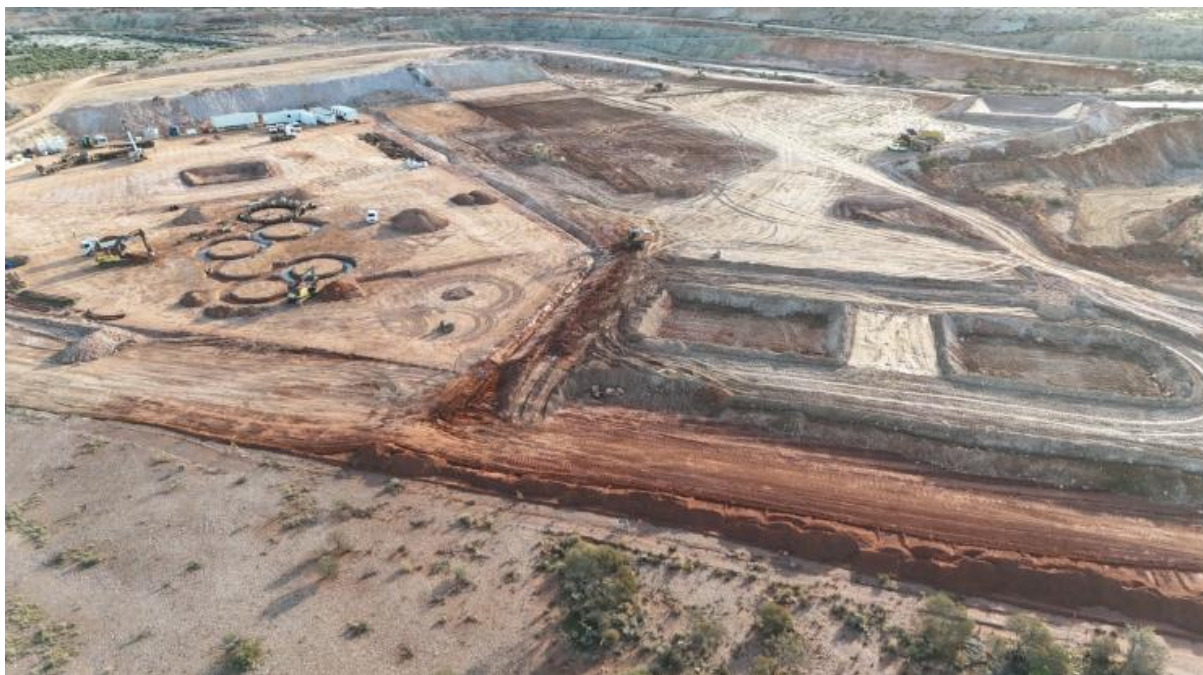
Figure 2 - Earthworks for the processing infrastructure (left) and the Process Water ponds (right) (28 June 2026)
