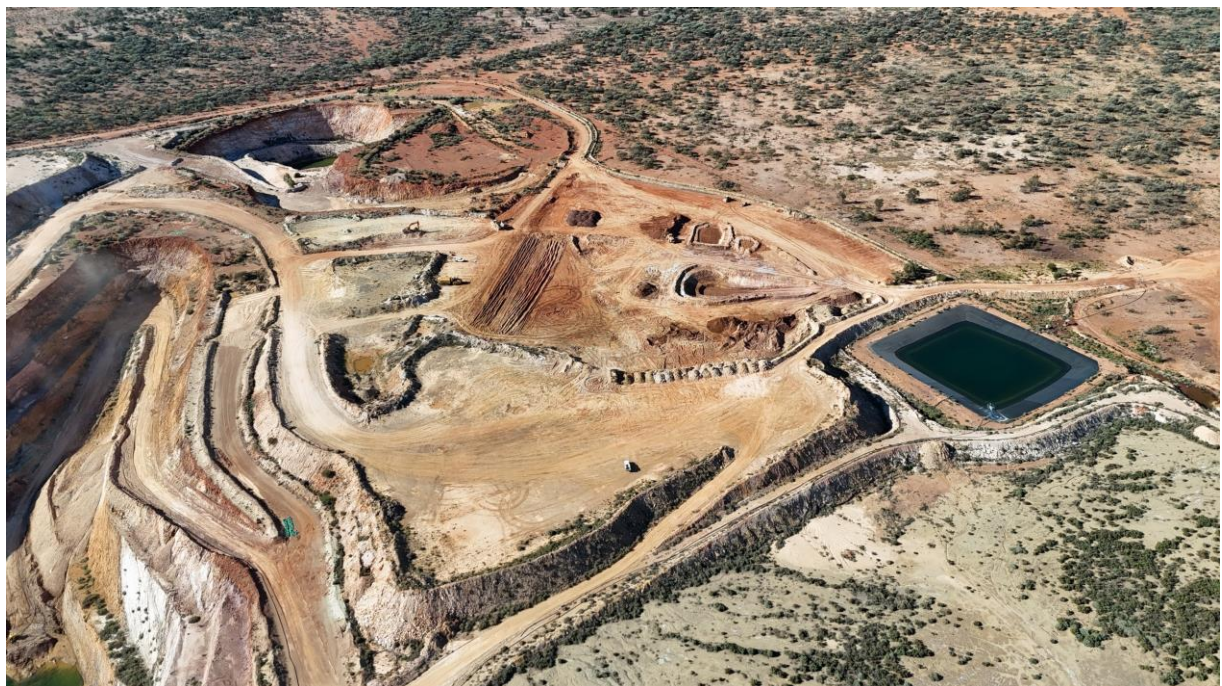
Figure 2 - Site remediation and establishment works underway (May 2026, pre-FID )
