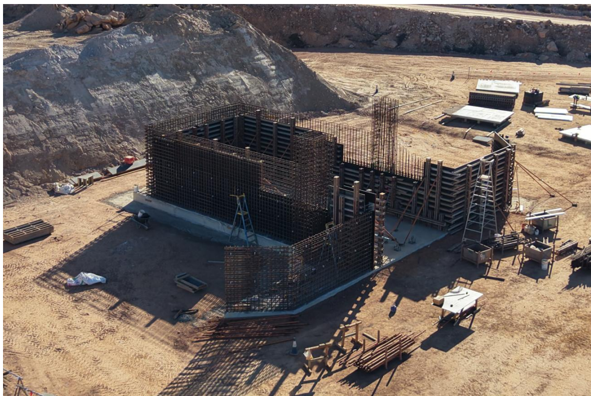
Figure 2 – Primary Crusher steelwork
