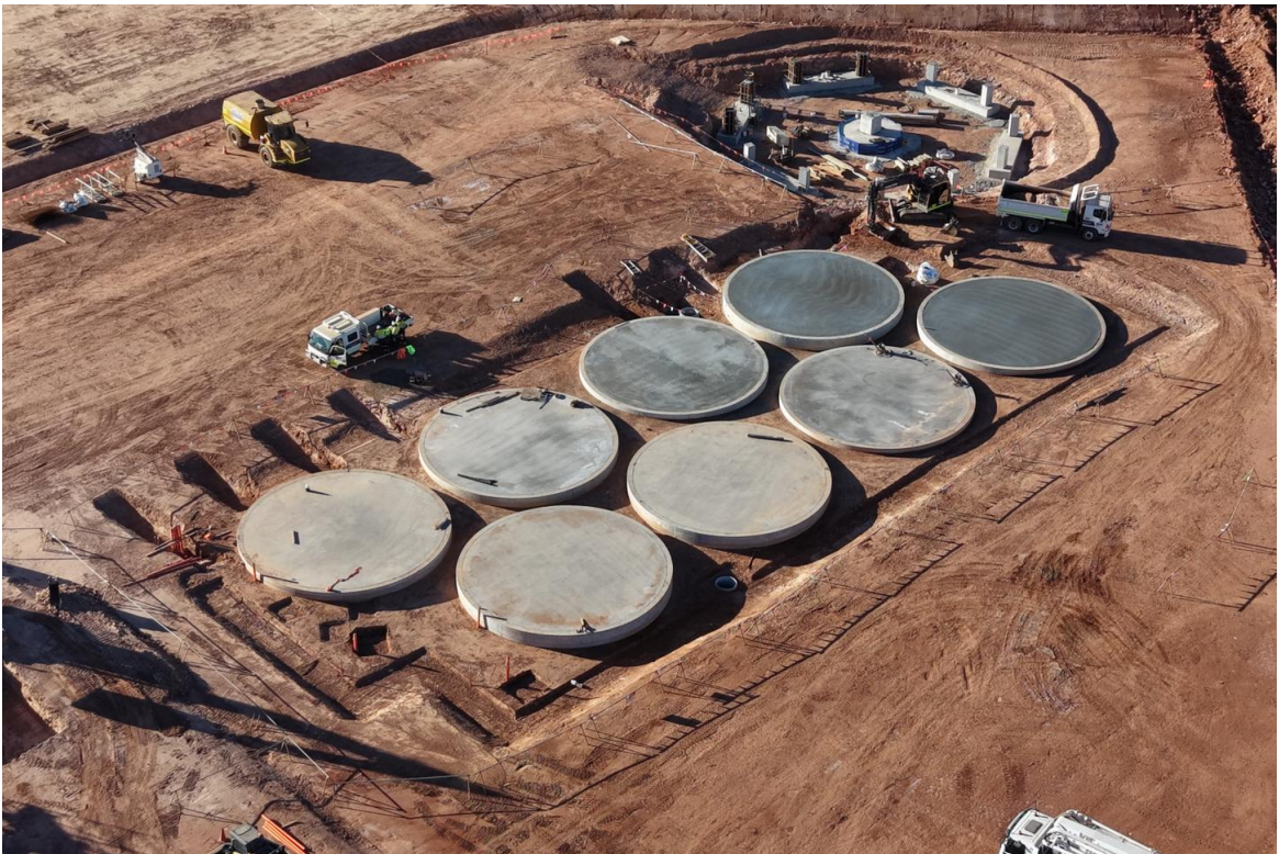
Figure 4 – CIL circuit and tailings thickener footings
