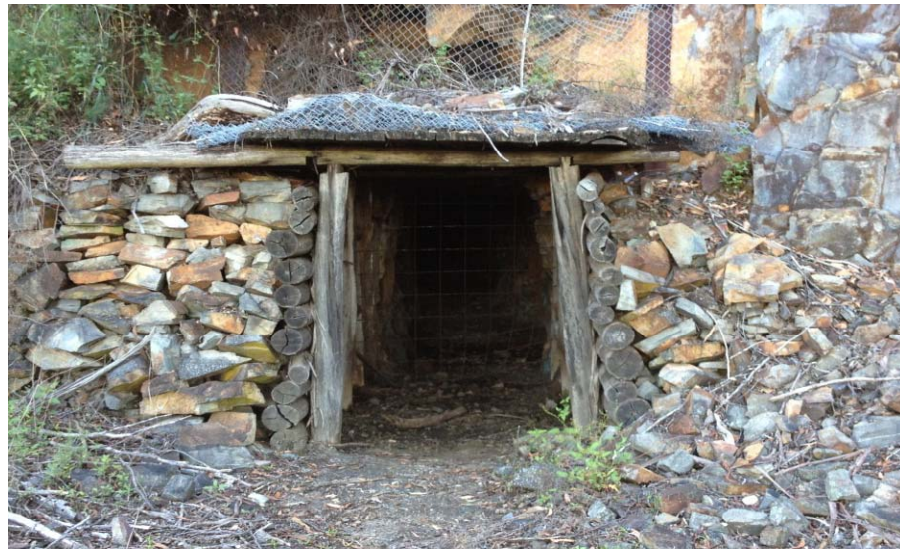
Northern Zone Adit completed in conjunction with PFS
