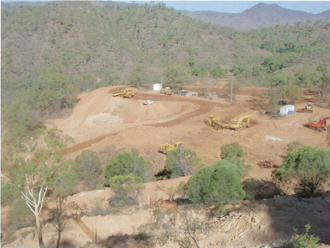
Earthmoving contractor's lay-down area in centre. Work commencing on Run-Of-Mine Ore Pad to left. Photo from north end of proposed initial pit, looking south-east – 27 November 2007.
