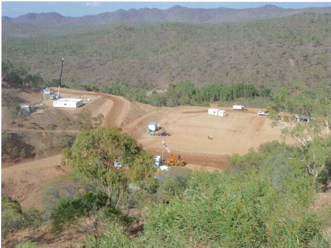
Processing plant foundations centre right. Site office building to left. Photo from north end of proposed initial pit, looking east – 27 November 2007.
