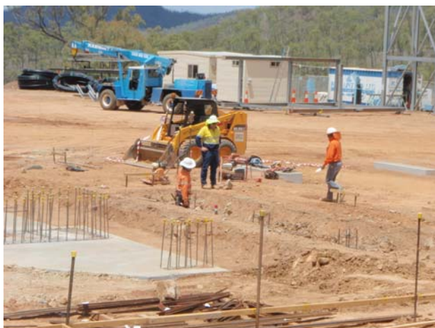
7 December 2007 – Concrete foundations progressing – GPB Construction at the Treatment Plant Site
