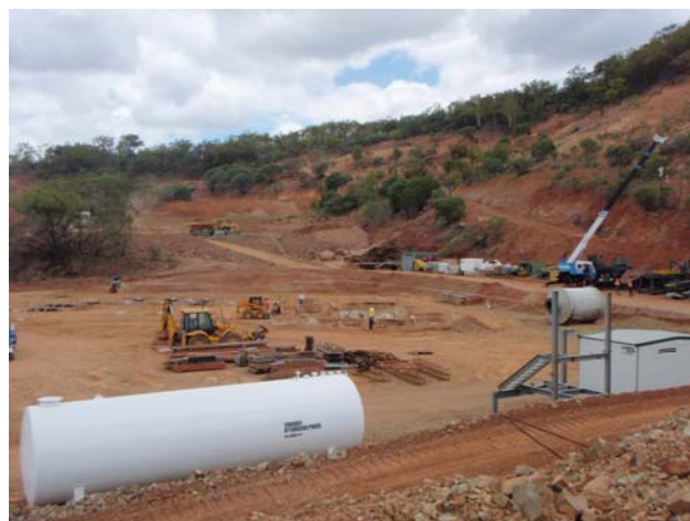
7 December 2007 – Initial concrete works in progress at the Treatment Plant Site
