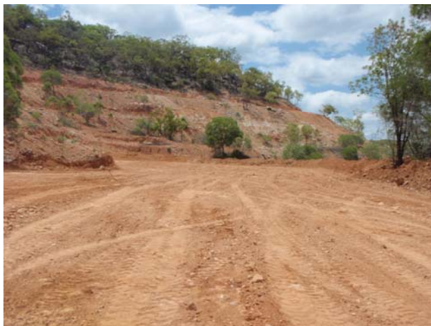
10 December 2007 – Initial earthworks on the main haul road
