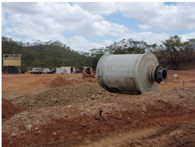
10 December 2007 – Ball Mill delivered to site
