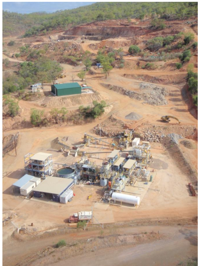
Aerial view of the Wolfram Camp processing plant with the open pit in the background
