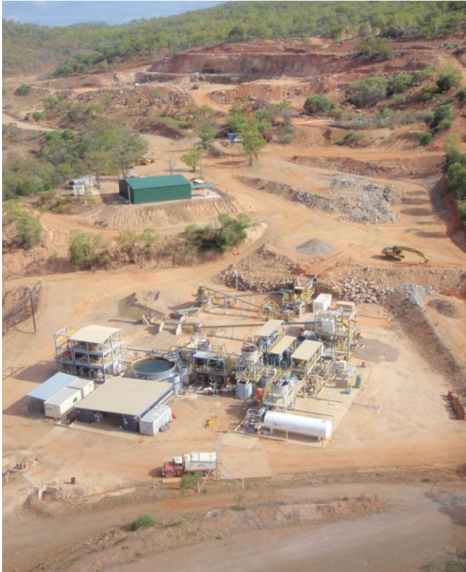
Wolfram Camp's existing 150,000tpa processing plant
