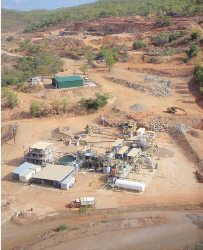
Wolfram Camp's existing 150,000tpa processing plant
