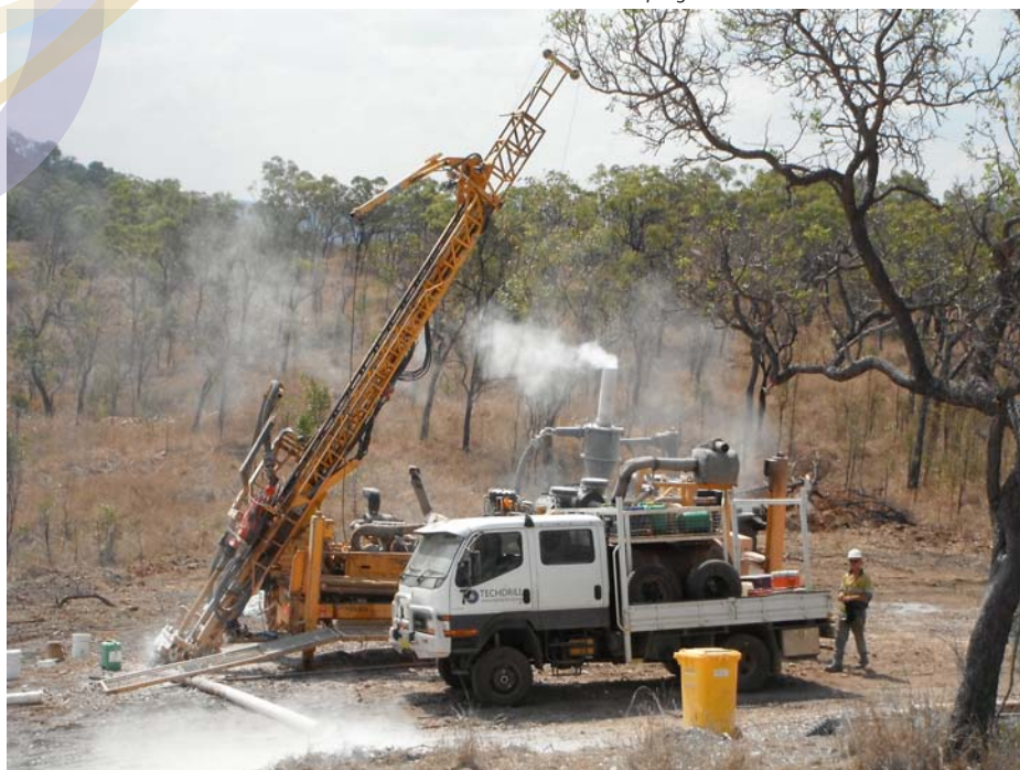
Mount Borium December 2012 Drilling
