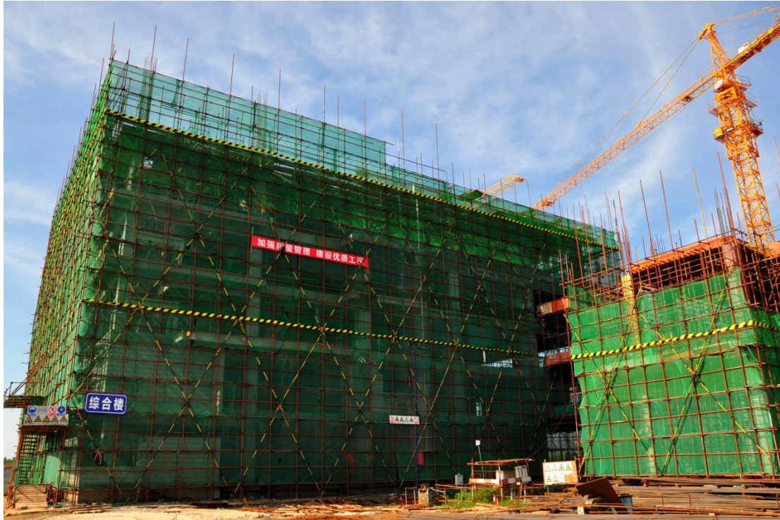
Image 3 – the Commercial and Administration Centre (taken on 24/09/14)
