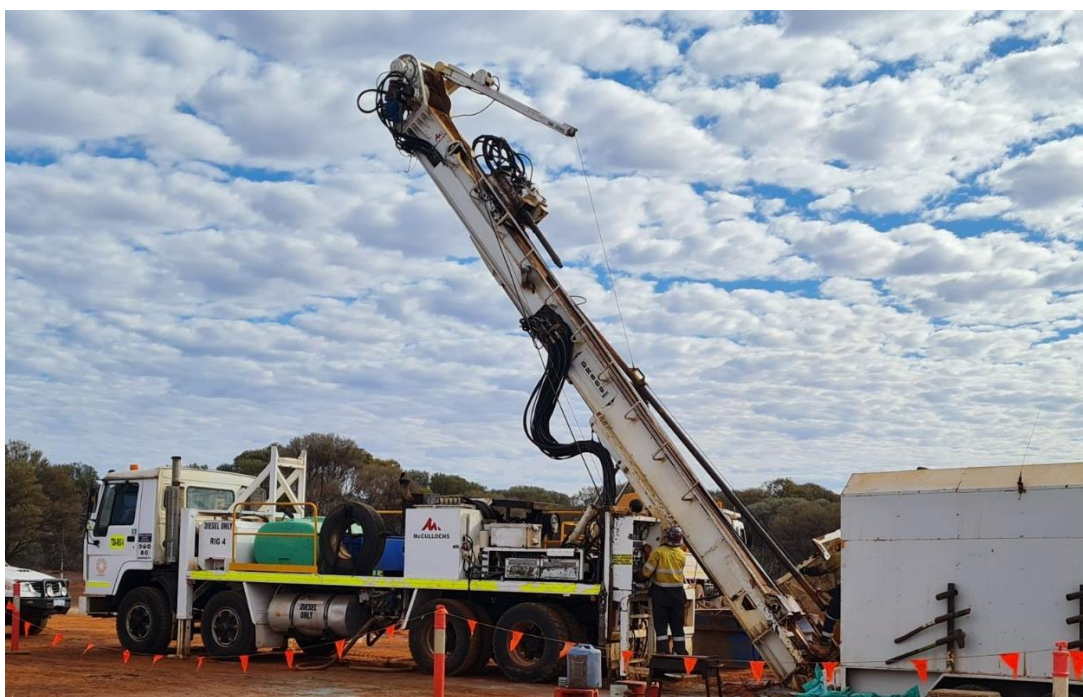
Figure 1: Topdrive diamond drilling at Kookynie Gold Project
