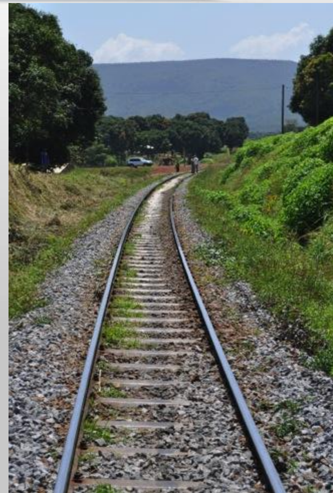
Rail line near the project area
