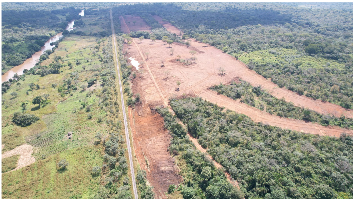
Image 4: Inland Rail Facility Earthworks
