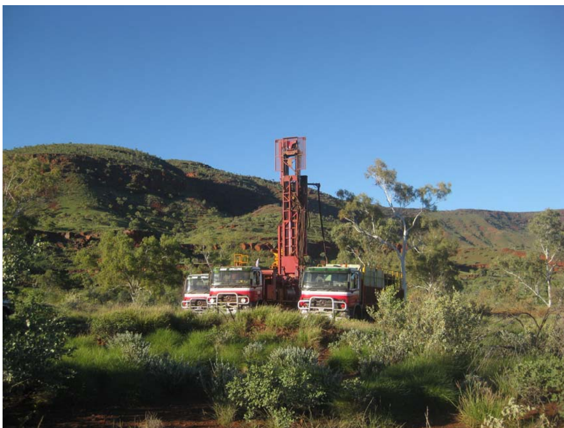
Drilling at the Winmar Deposit, April 2011.
