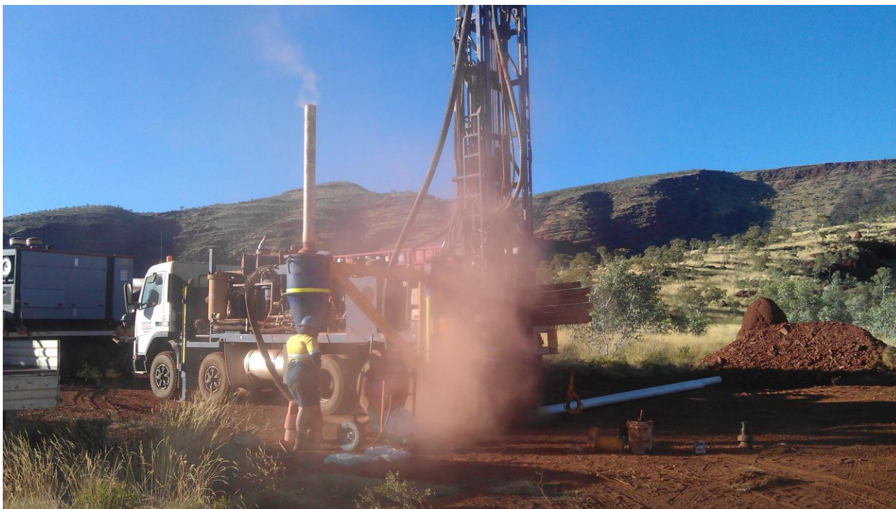
The next phase of drilling underway at Winmar's Hamersley Iron Project
