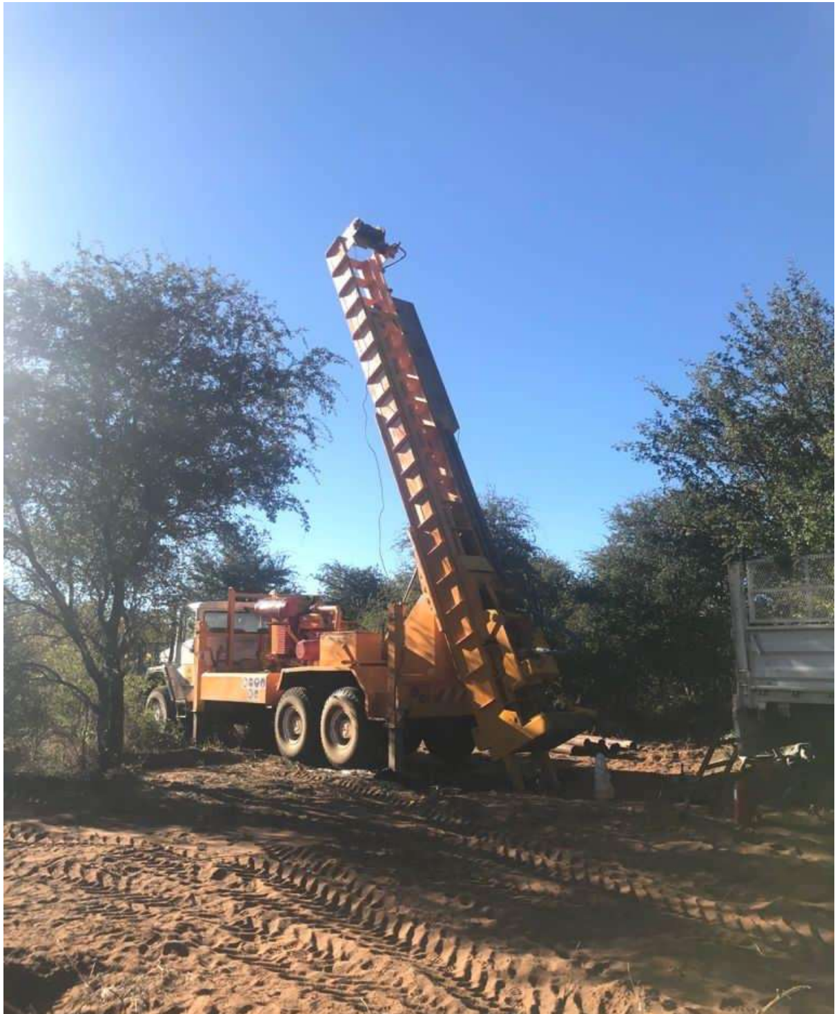
Figure 2. RC rig testing targets on the Endurance Prospect.
