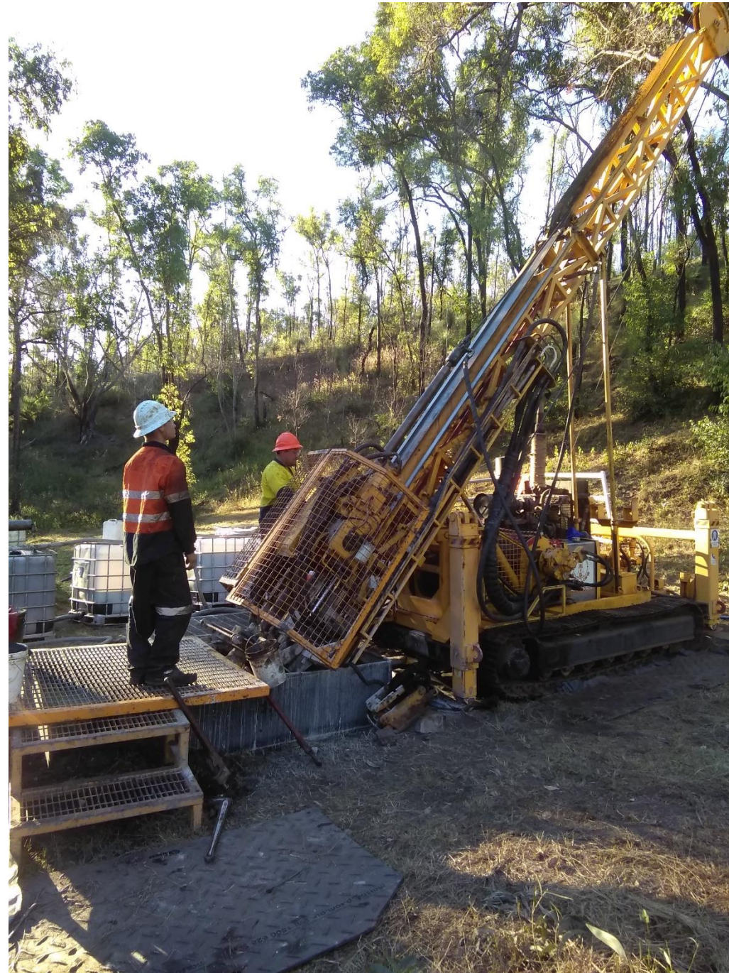
BD019-001 Drill Site Briggs Copper Project Queensland
