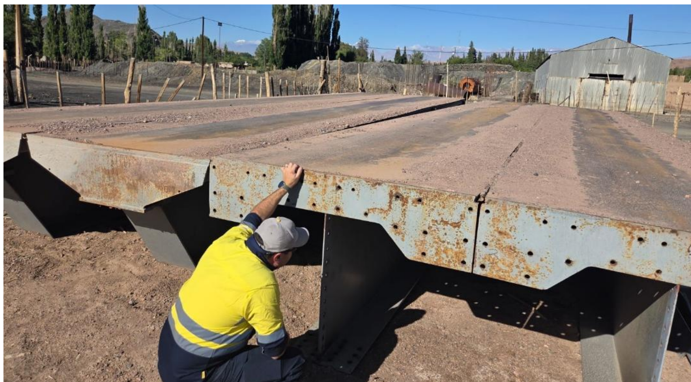
Figure 6 - Bailey Bridge Module Segments Inspection
