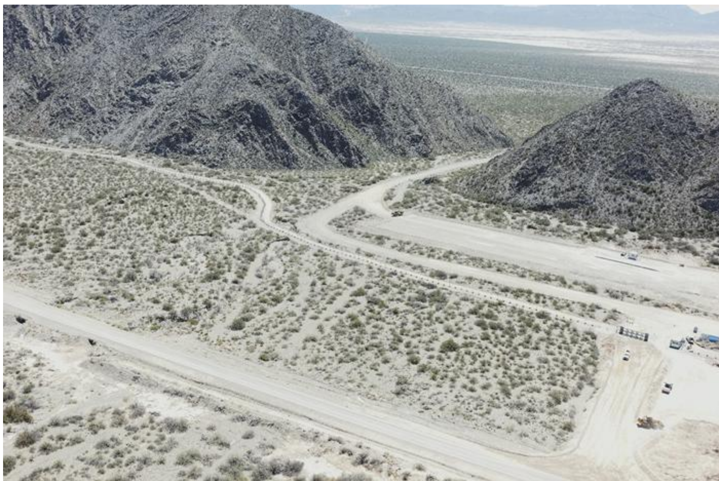
Figure 10- Main Access Gate as at 17 December 2025
