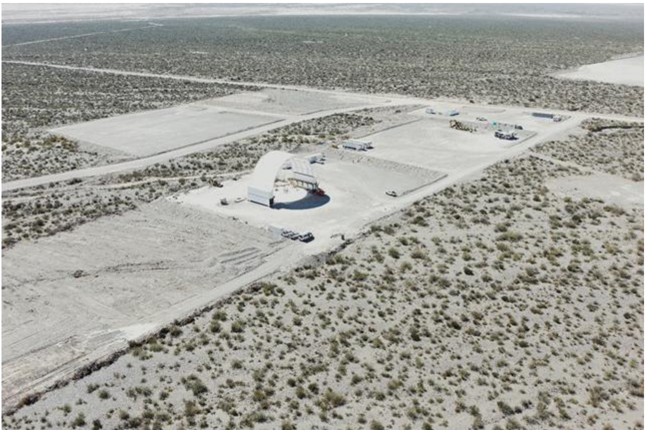
Figure 8 - Site Infrastructure Development as at 17 December 2025
