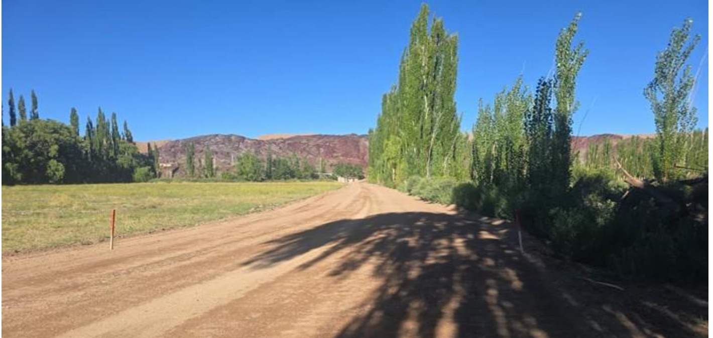
Figure 4 – Completed segment of Calingasta Bypass Road
