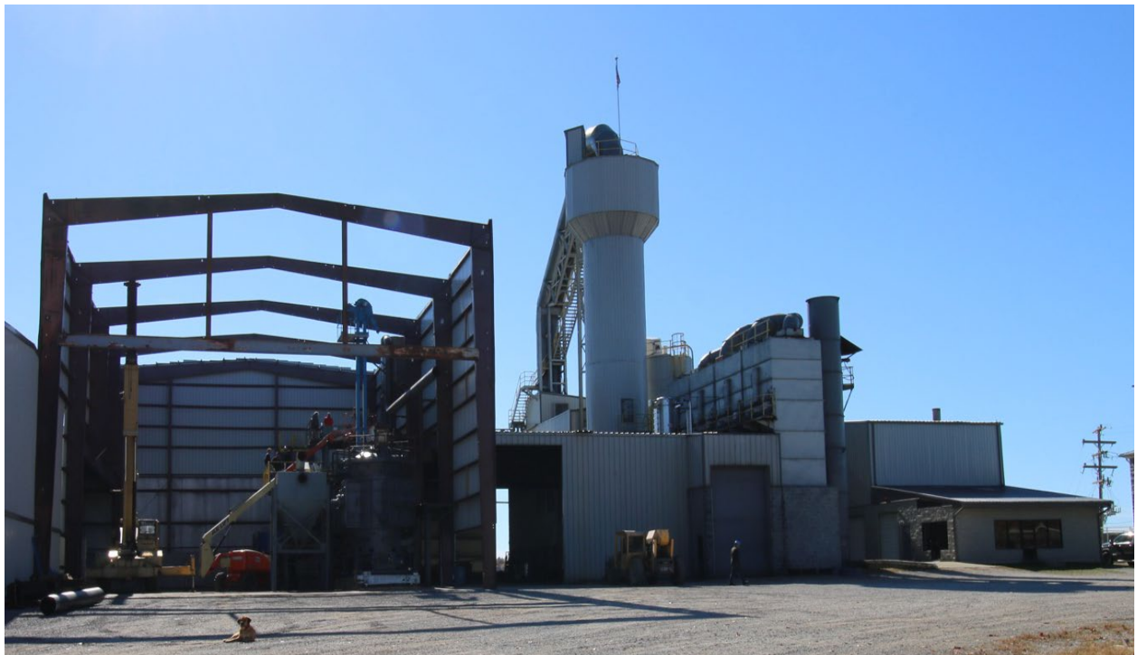
Figure 2: Front view of the Facility
