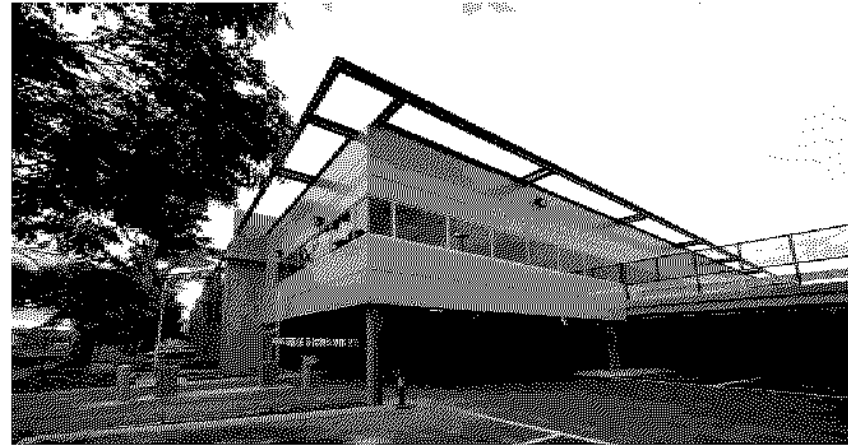
Toll Priority, Douglas Street, Port Melbourne, VIC Completed in 2006 with an approximate value of $19.0m Developed in joint venture with Australand Acquired by Australand
