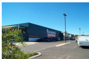
Bunnings Kalgoorlie, Western Australia (100% Interest)
