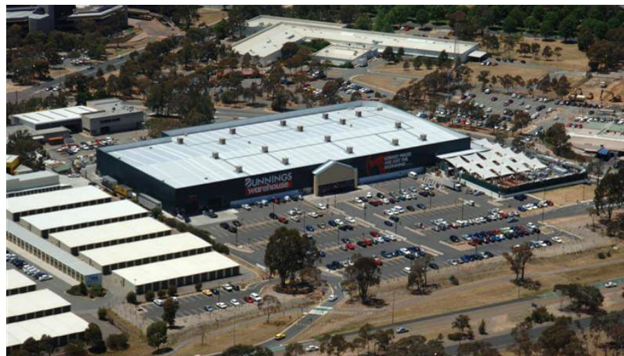
Bunnings Belconnen, part of the $130m Bunnings portfolio acquired in June 2006
