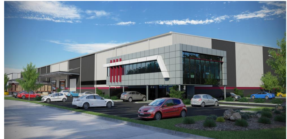
Axima Logistics – Smithfield Distribution Facility
