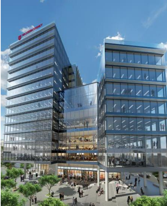
1PSQ, Western Sydney University, Parramatta – Completed
