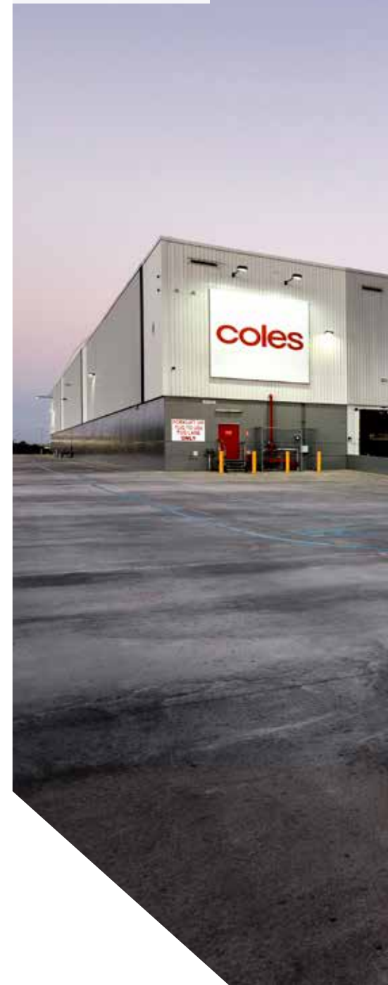
Coles Distribution Centre WA
