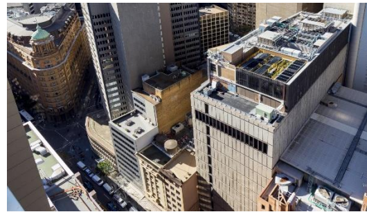
Telstra Exchange, 76-78 Pitt Street, Sydney
