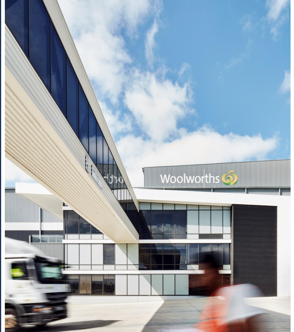
Woolworths, Distribution Centre, Dandenong
