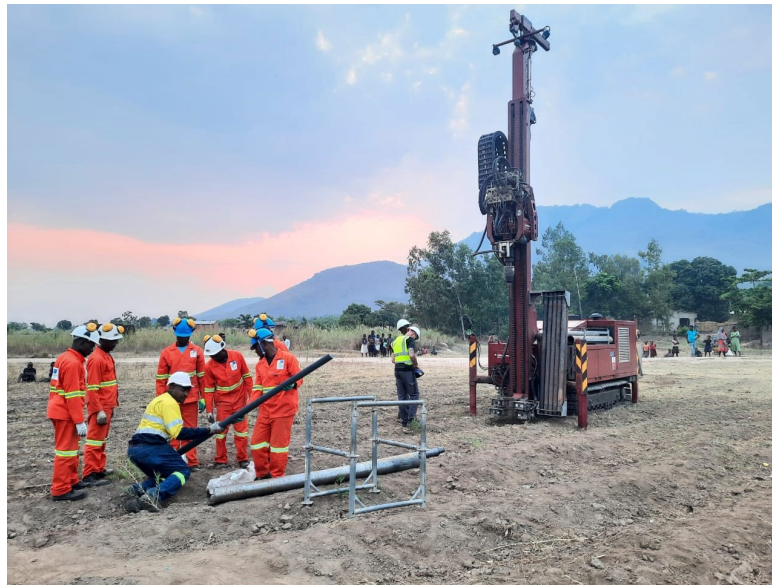
Figure 2 Sonic Rig Drilling Hole No.1
