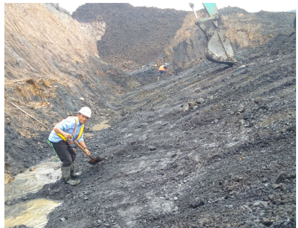
Cleaning the Coal Seam Roof
