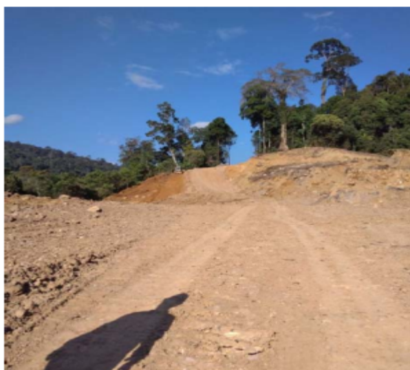
Sealed Haul Road Completed
