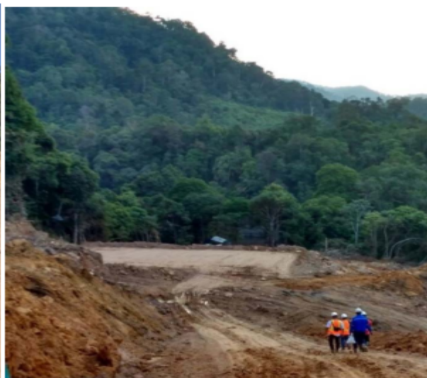
Sealed Stockpile Pad Completed
