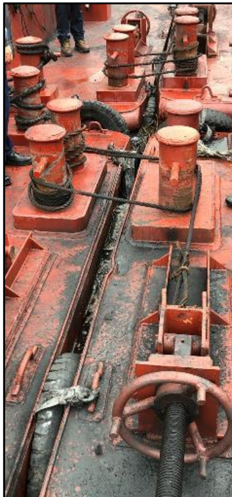
Joining Four Barges
