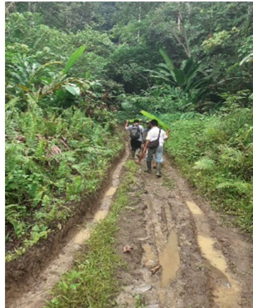
Cleared Road Prior to Forming and Sealing
