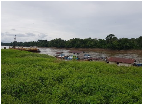
Bomban Jetty on the Barito River
