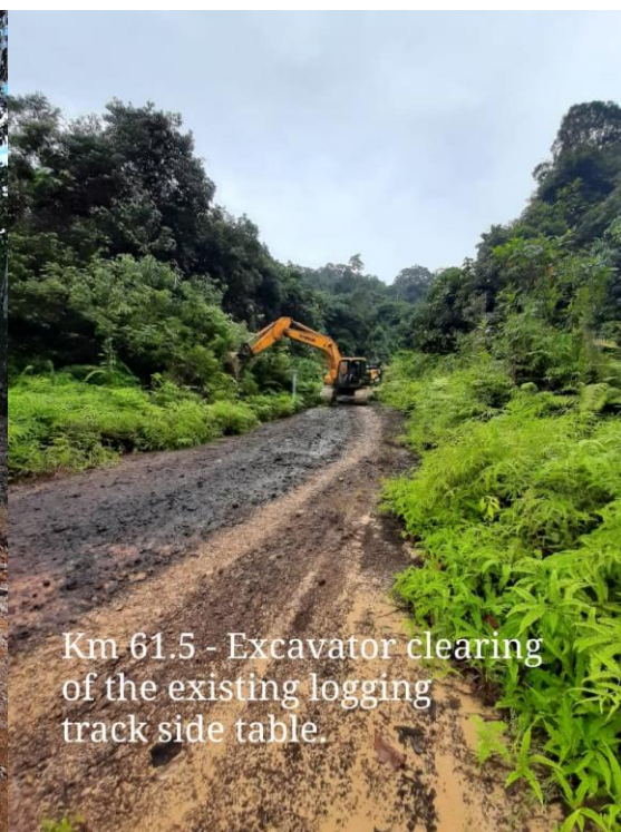
Km 56 - blue arrow shown finished road sub-base. Green arrow indicates the bund at backfill area to prevent erosion on the road.
