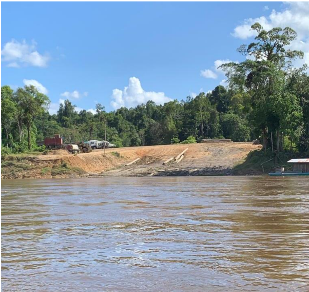
Krajan Jetty Development
