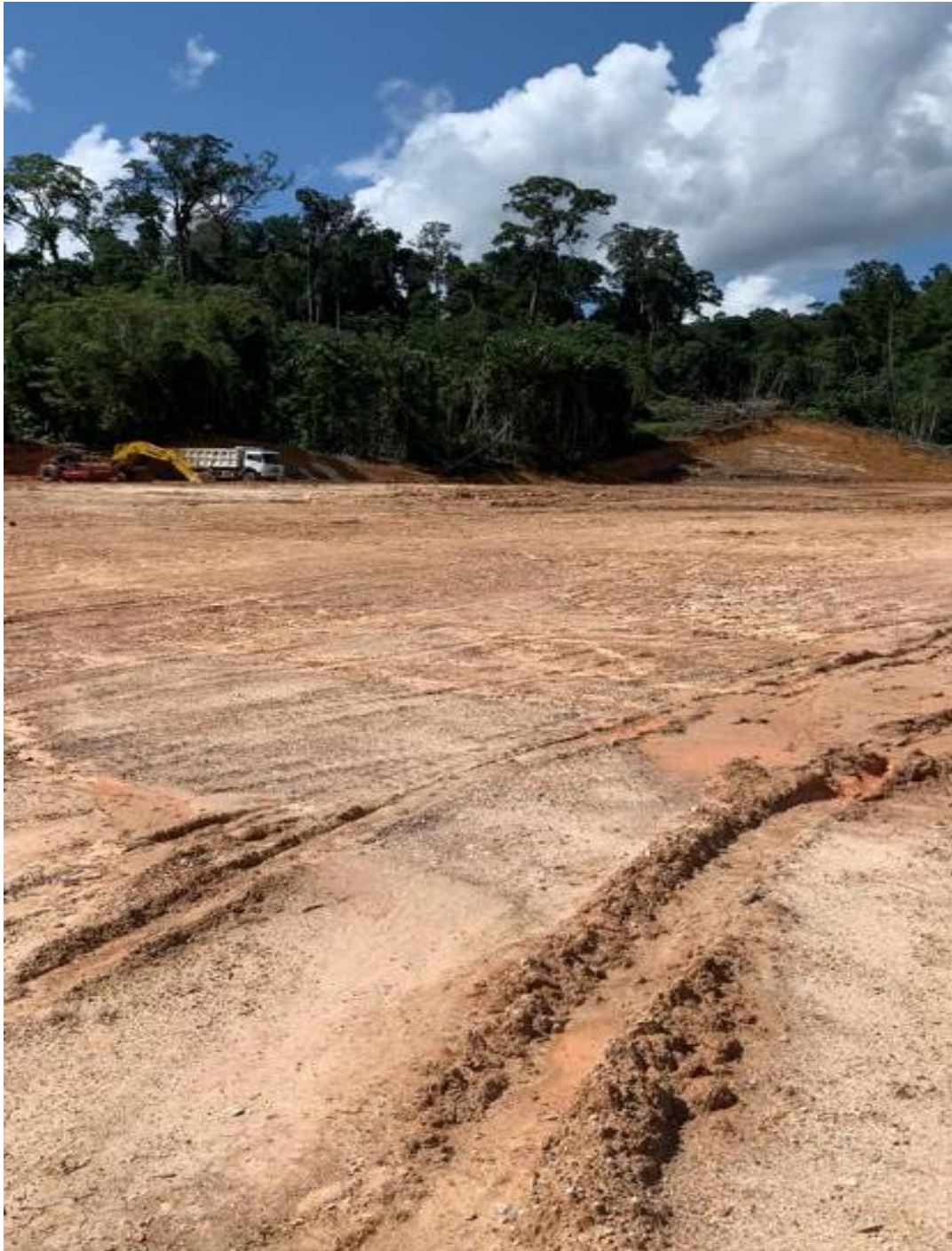
Coal stockpile area development at Krajan Jetty
