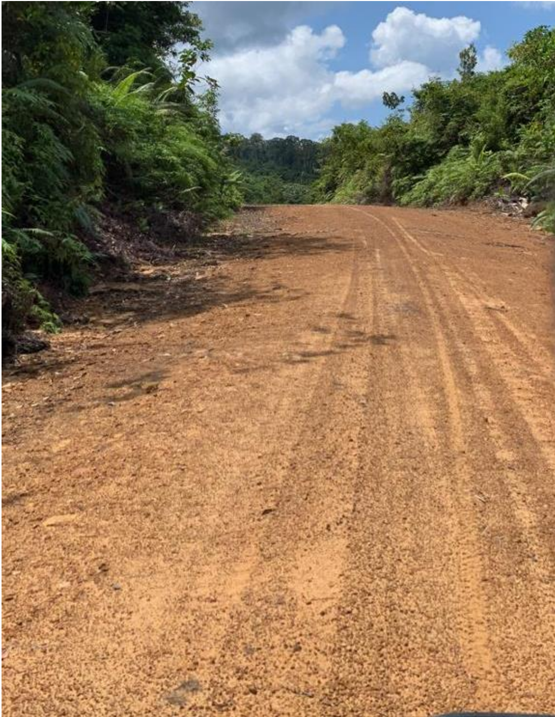
Haul road construction
