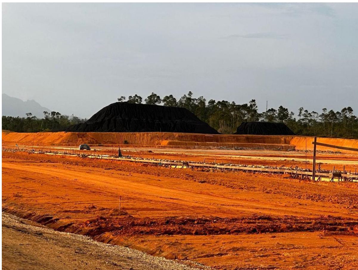
Coal Stockpile at Batu Tuhup Jetty
