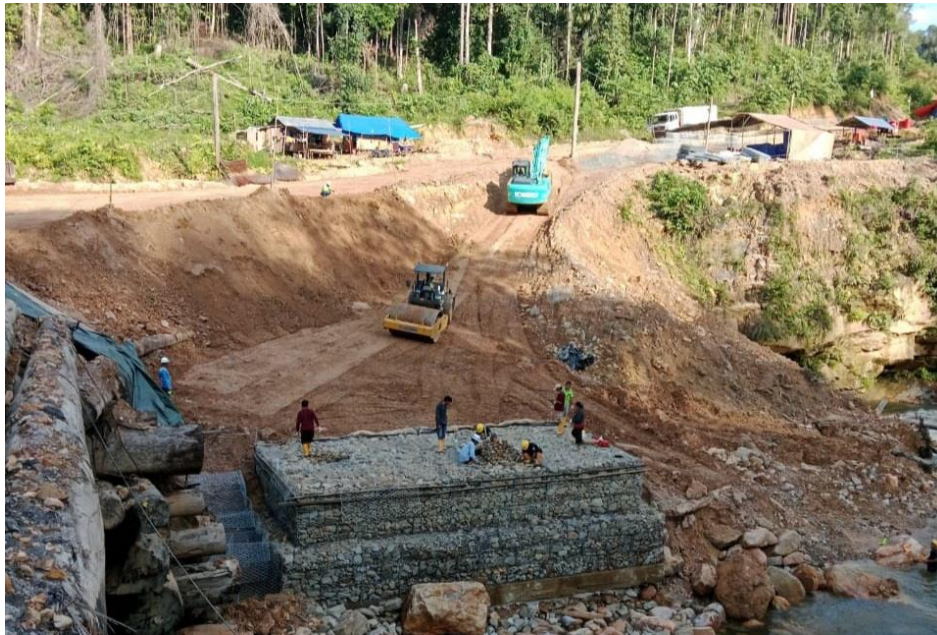
Mohing Bridge Construction Progress
