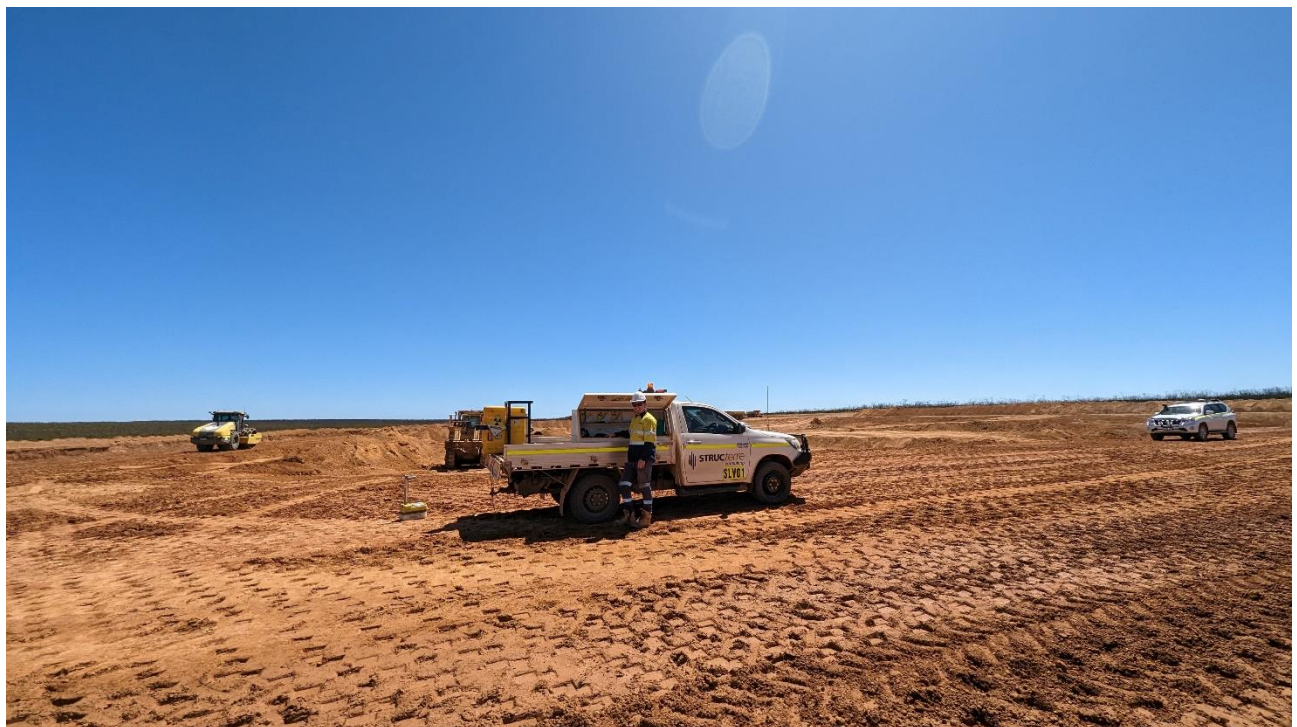
Figure 2: REC Consultants managing construction of TSF.
