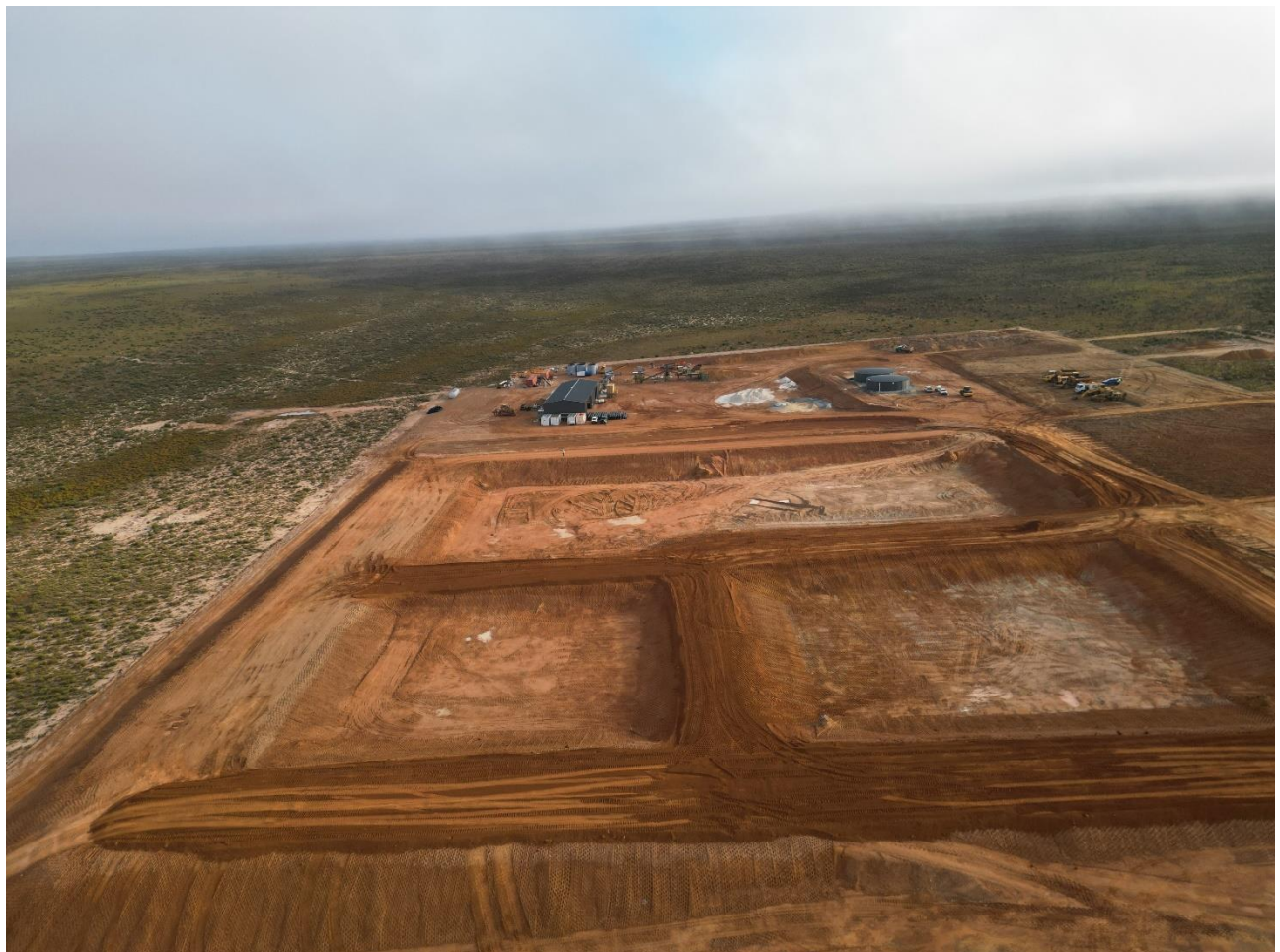
Figure 1: Kat Gap Processing Facility showing TSF progress.
