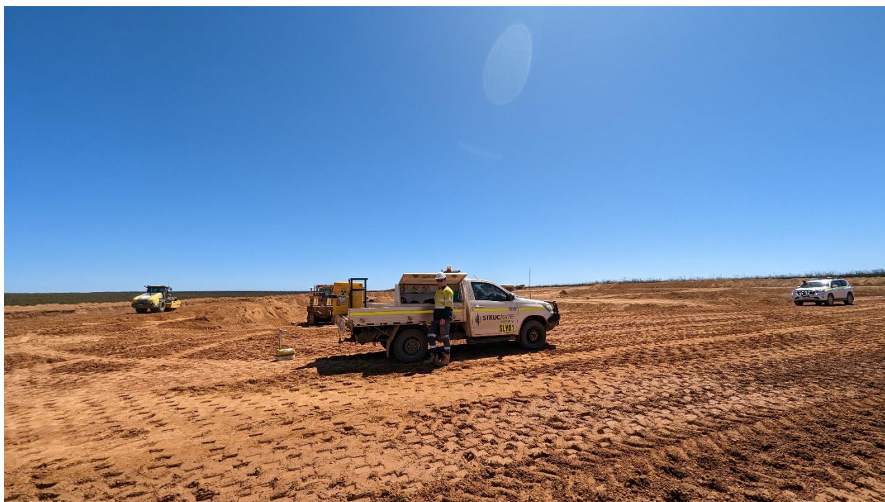
Figure 2: REC Consultants onsite managing the construction of TSF.
