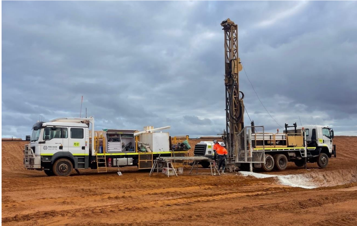
Figure 2 & 3: Kat Gap Tailings storage facility – Drilling of diamond hole for VWP installation.
