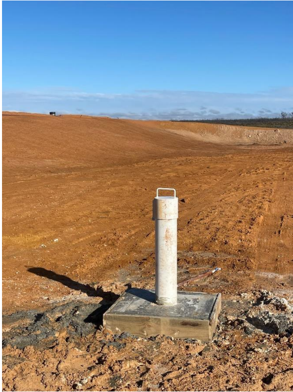
Figure 4-7: Kat Gap Monitoring Bores completed and capped.
