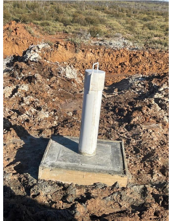
Figure 4-7: Kat Gap Monitoring Bores completed and capped.
