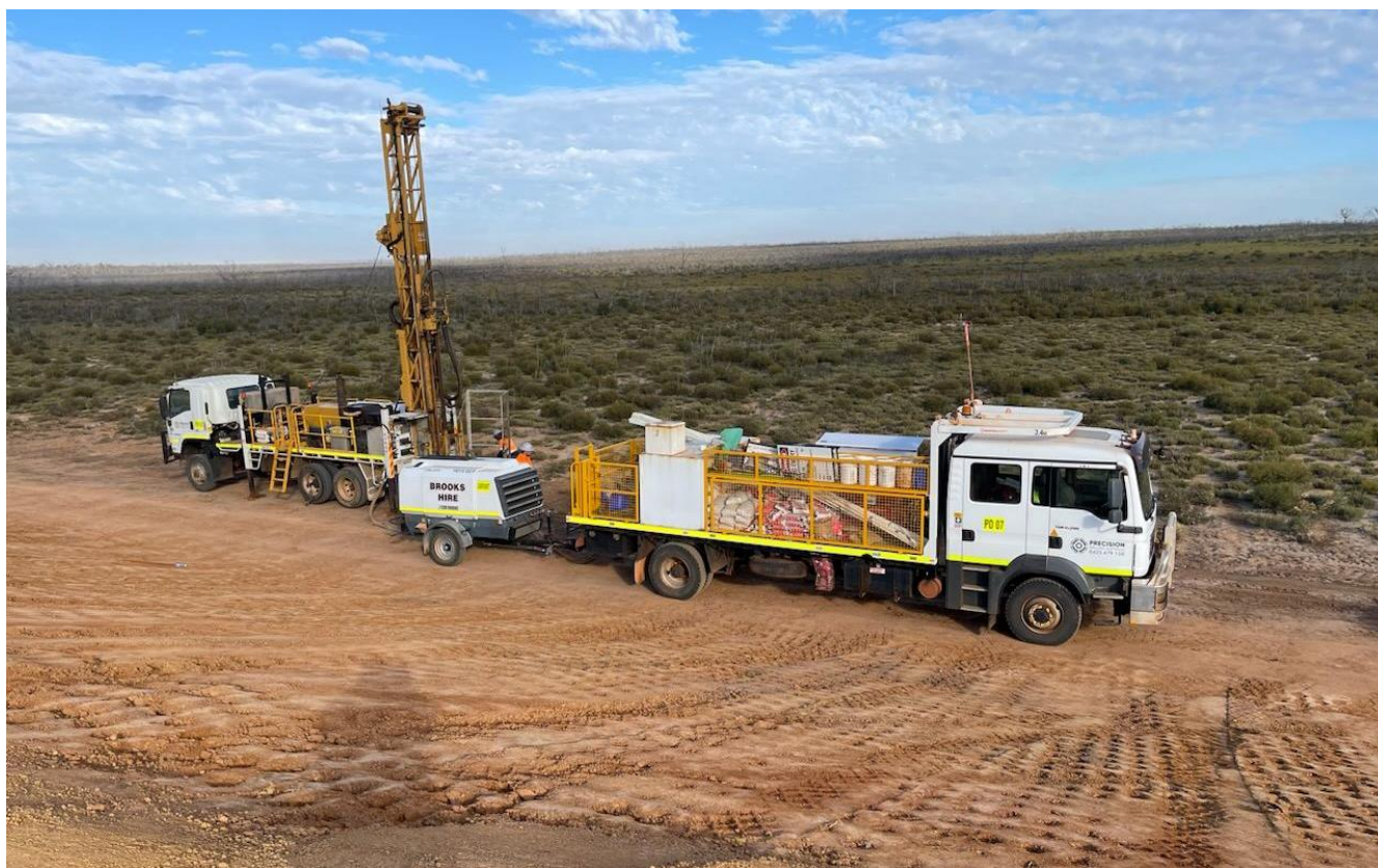
Figure 1: Kat Gap Tailings storage facility - VWP Installation.
