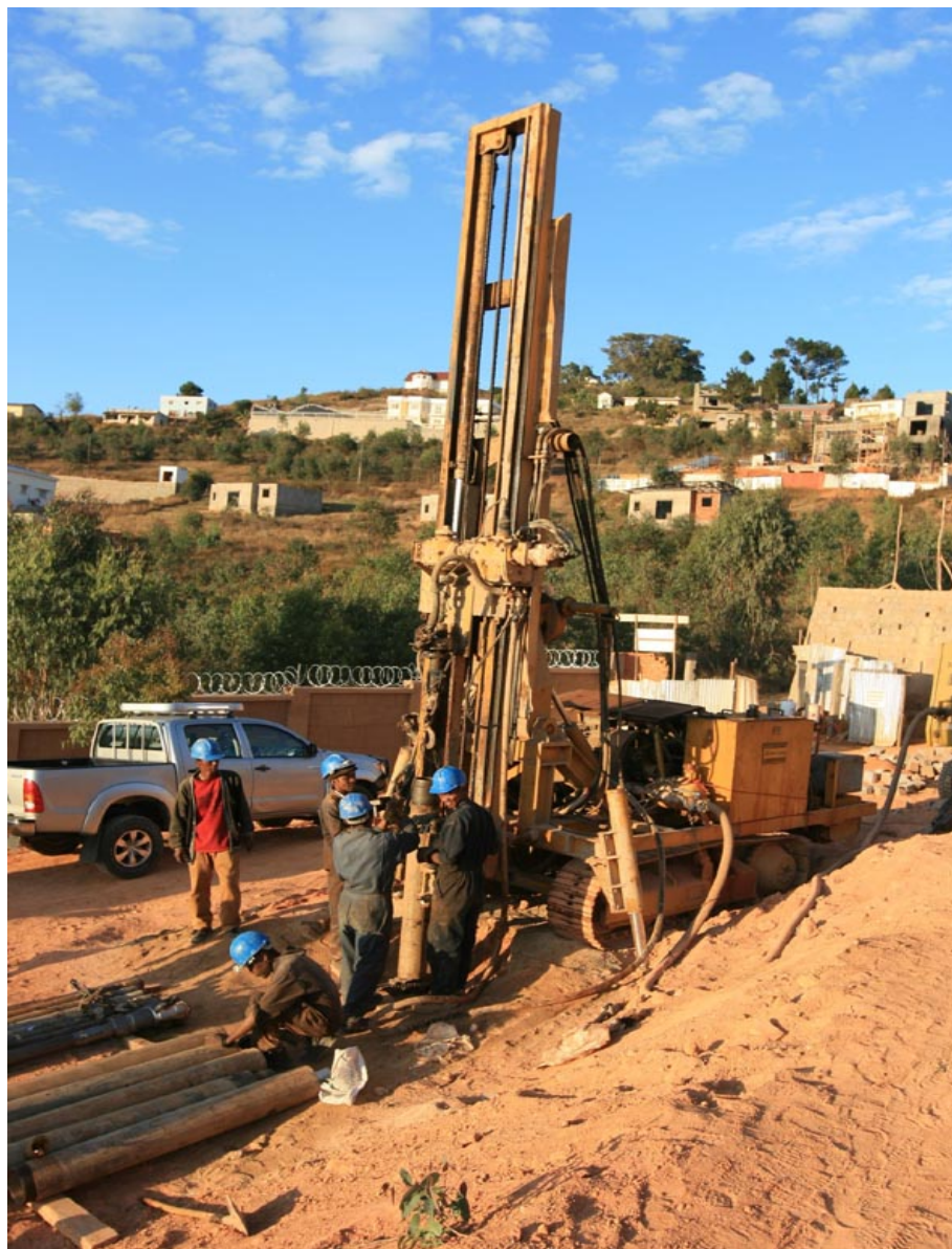
Atlas Copco drill completing a domestic water bore in Antananarivo
