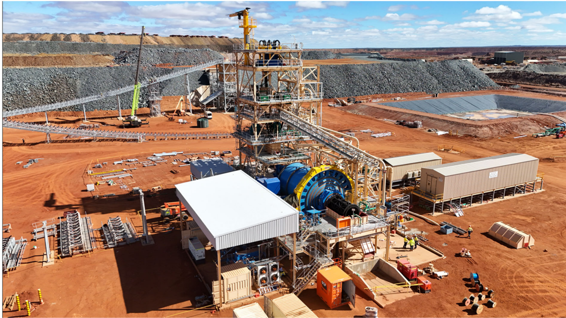
Karlawinda Expansion Project – Mill area nearing completion.
