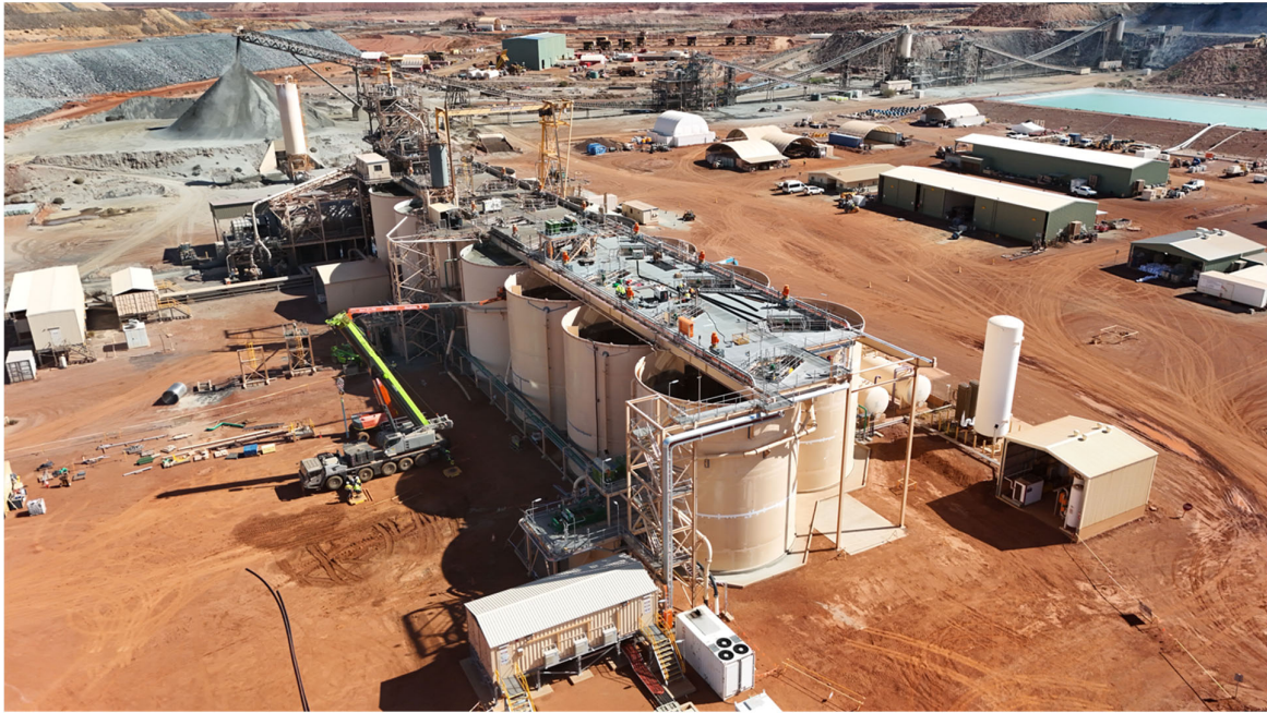
Karlawinda Expansion Project – CIL circuit extension with top of tank steel sections in place.
