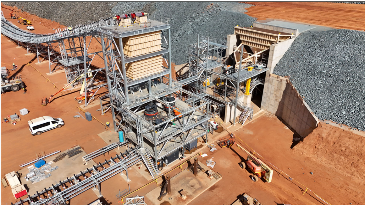
Karlawinda Expansion Project – Primary/Secondary/Tertiary crusher building and ROM 2.
