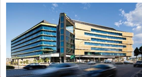
Energex House – Cromwell Riverpark Trust
