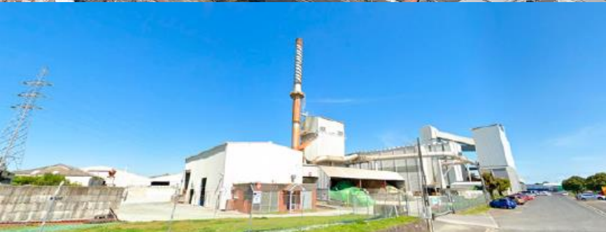
VISY FACILITY, PENROSE, AUCKLAND, NEW ZEALAND
