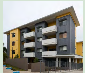
45 PENDLEBURY ROAD, CARDIFF, NEWCASTLE
