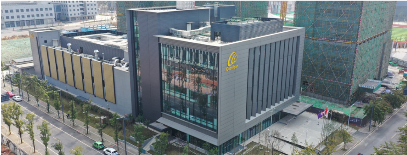
Our new manufacturing facility in Chengdu, China.
