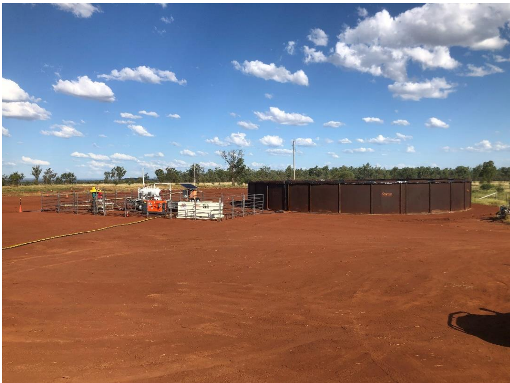
Figure 2: Mahalo North 1 well pad with water storage tanks and well test facilities installed, where the production test has recently commenced.
