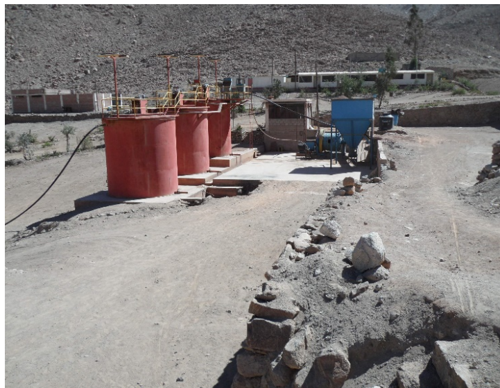
Figure 16: “Existing leach tanks: with accommodation block at rear left & Laboratory in the background: Chimu Gold Plant”
