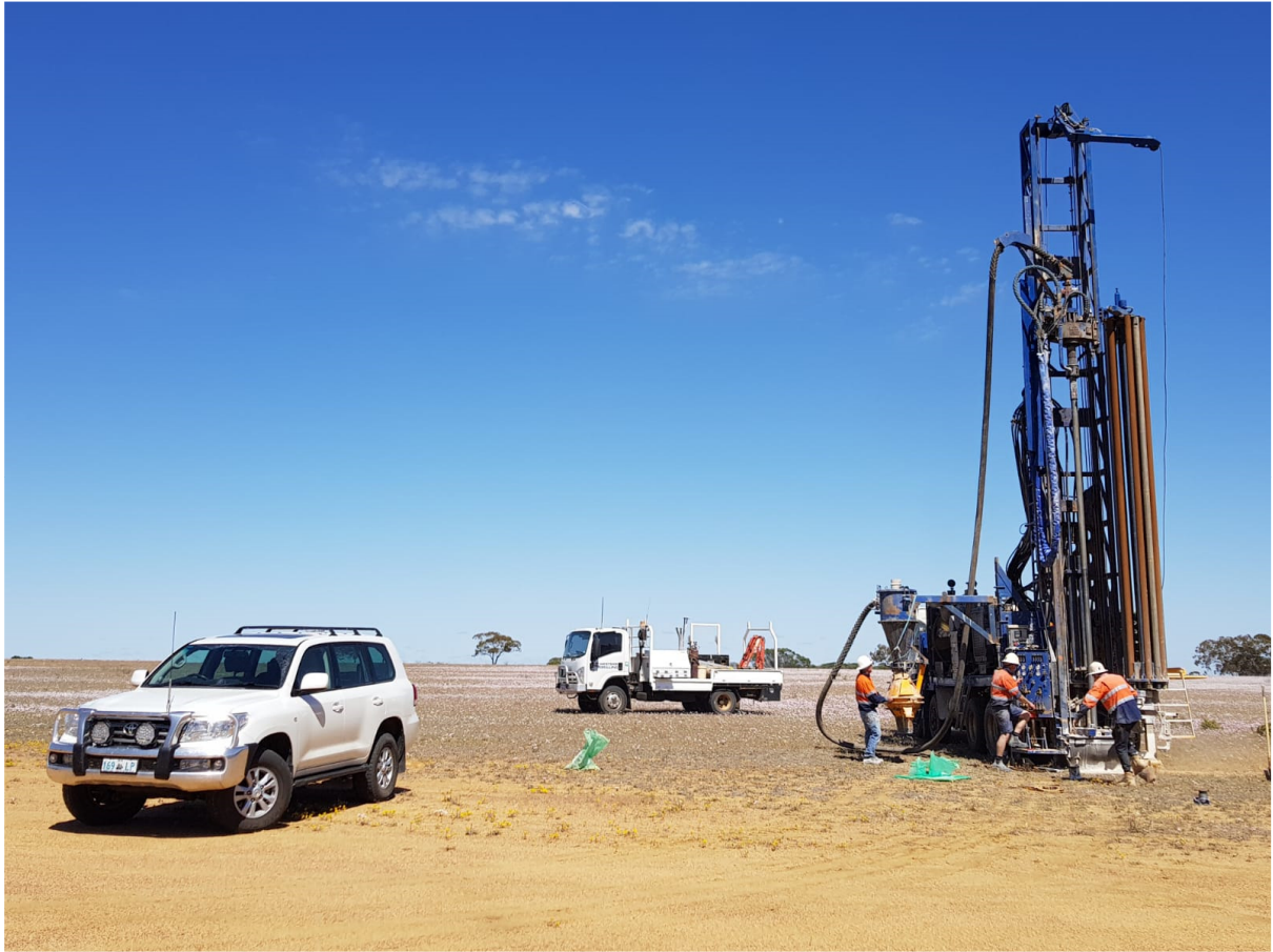
Figure 1 - 2019 Water Bore Air-core drilling program.
